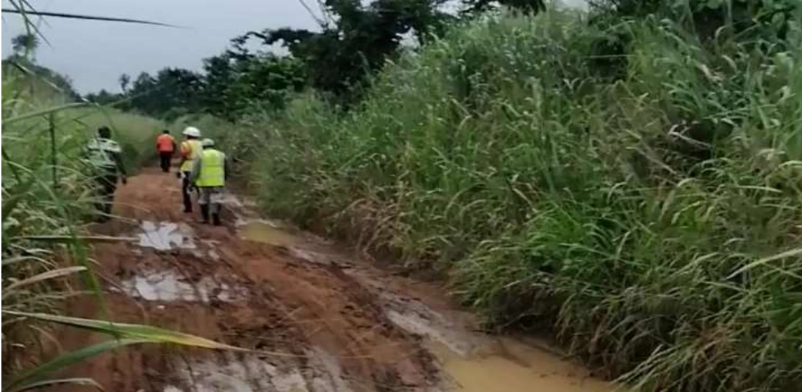
Plate 3-2: The other access route to project site between the GRIDCo 161 kv line and NVTI structures (left side of substation)
