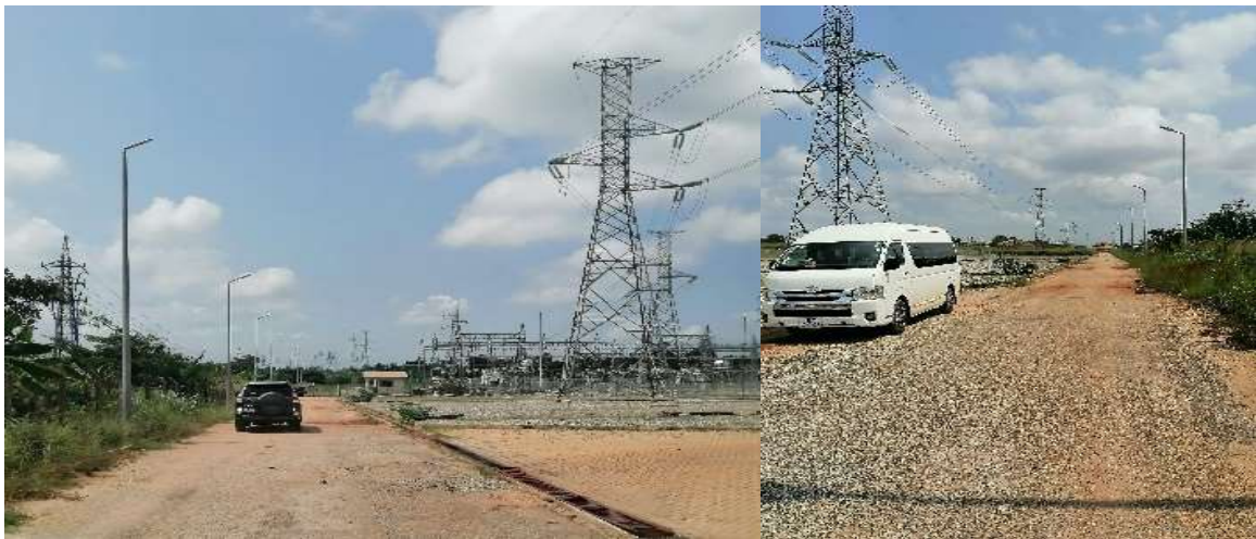
Plate 3-1: One access route to project site along the GRIDCo 330 kV Substation (right side of substation)
