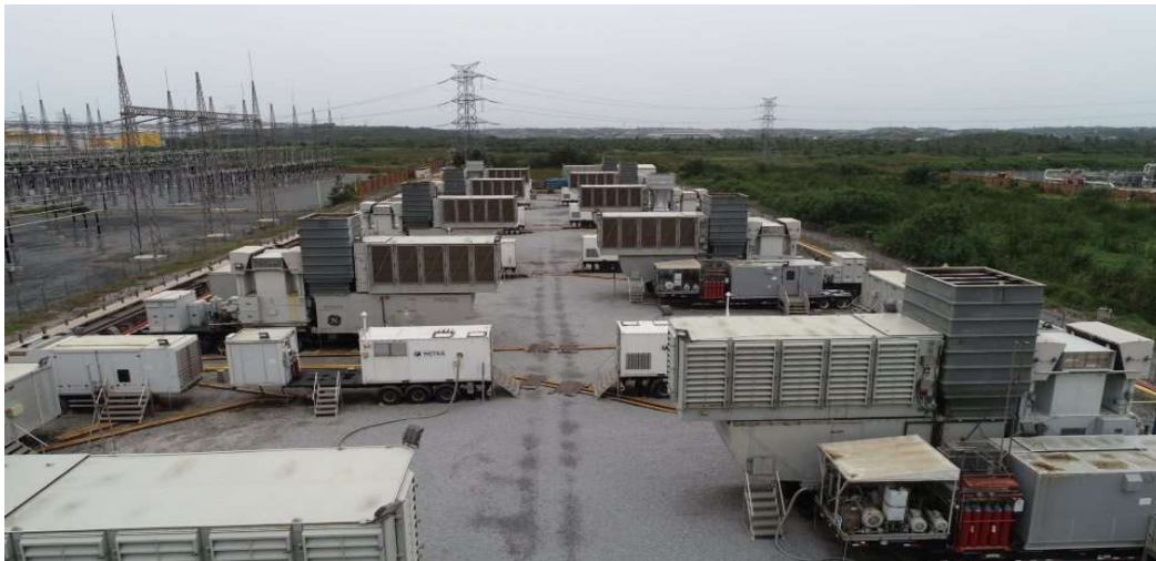
AMERI Power Plant - Gas Turbine Island and Associated Balance of Plant at Aboadze, near Takoradi
