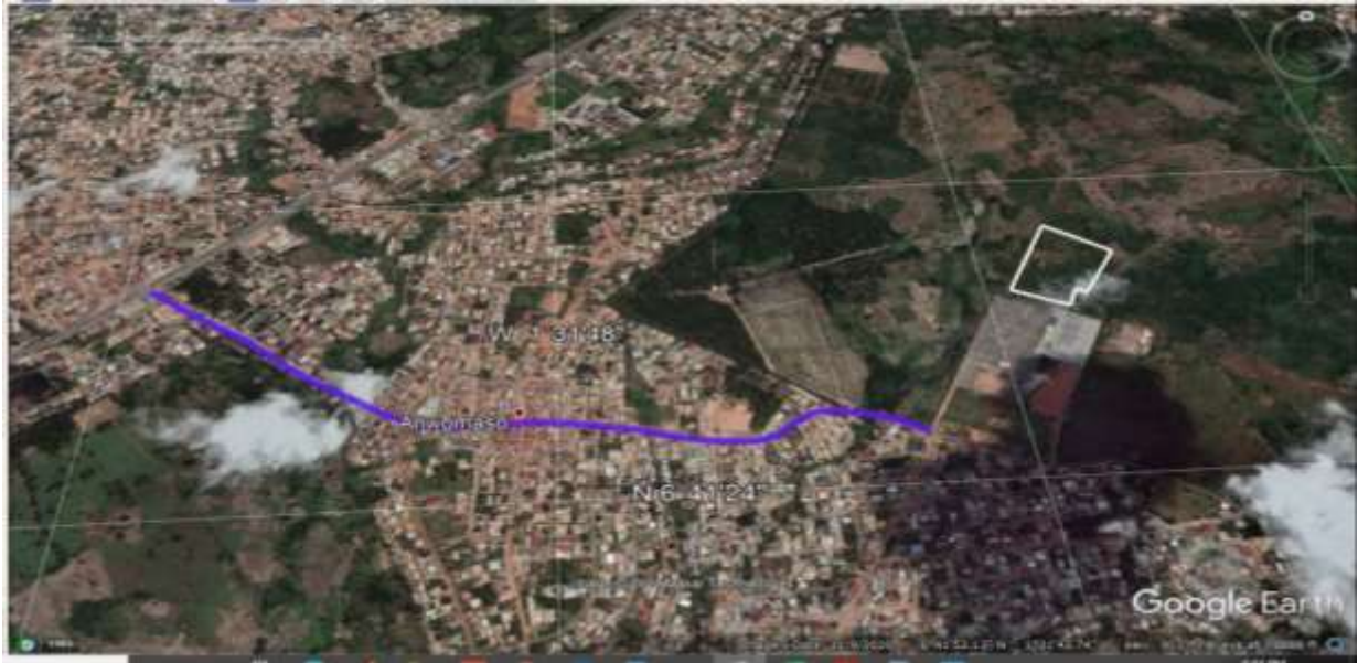
The Main Access Road from the Ejisu - Kumasi Highway
